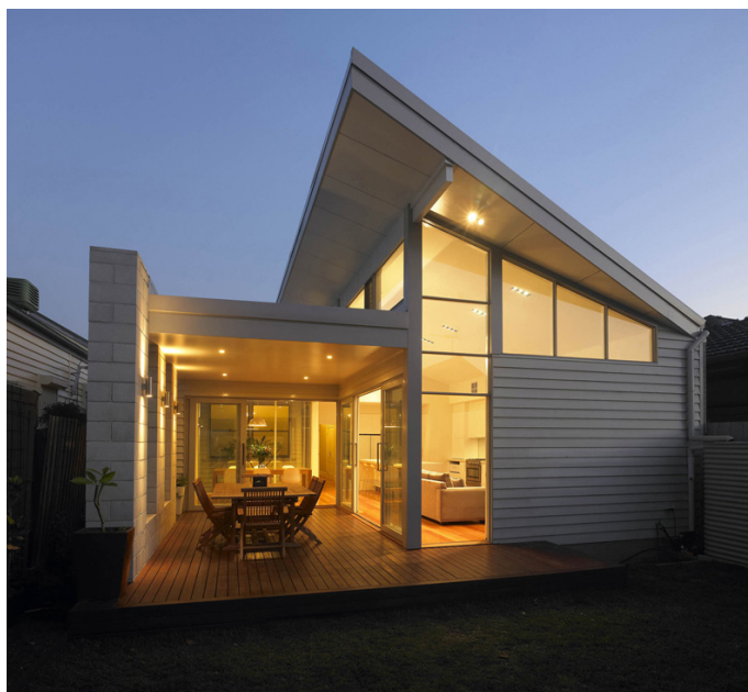
Skillion roof and extended north facing windows improve passive heating during cooler months.
